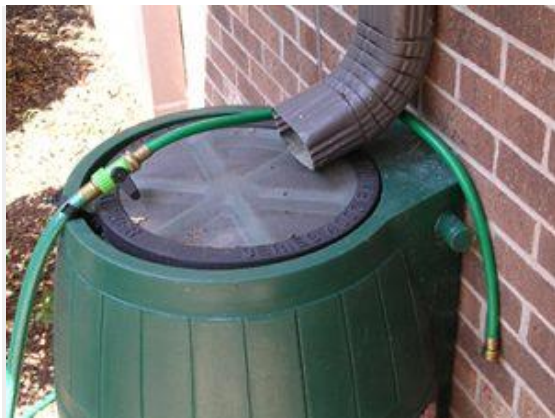
Keep rain barrels screened to exclude debris and mosquitoes. (Photo – M. Waldvogel, NCSU)
